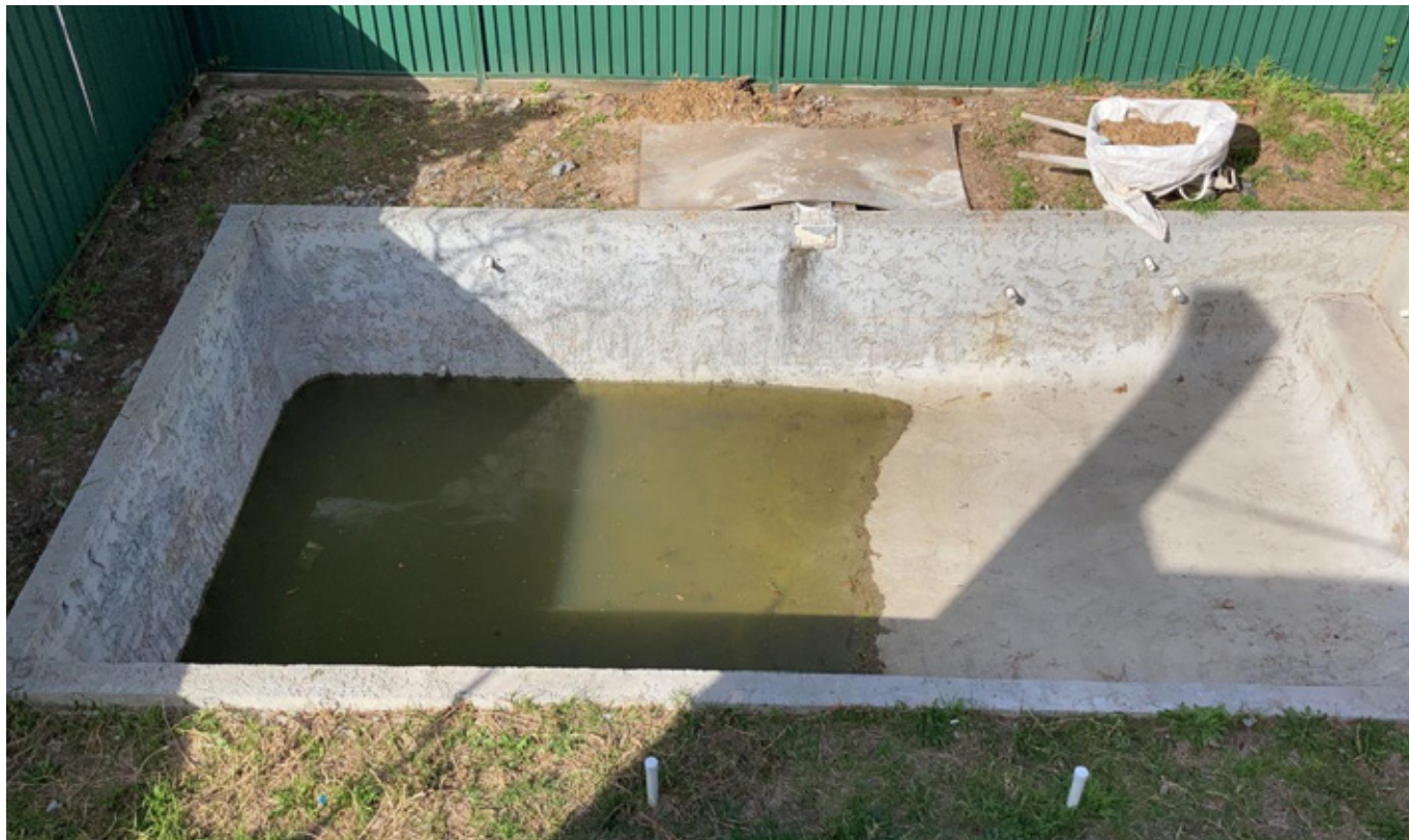
CONCRETE POOL SHELL BEFORE SEALING
