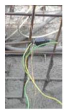
These shall be connected by an Equipotential Bonding conductor to the electrical earthing system of the property.
